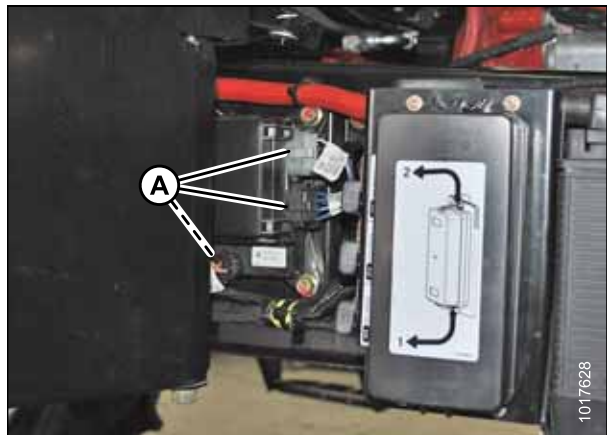
Figure 1.19: Chassis Relay Module
