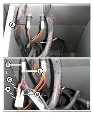
Figure 3.100: Single Connector Hookup Top - Before Connecting the Switch Harness Bottom - After Connecting the Switch Harness
