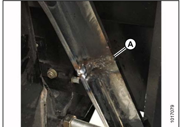
Figure 3.7: RH Brace with Groove Filled with Weld
