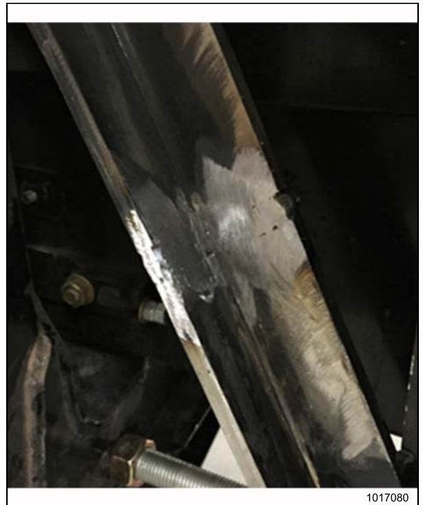
Figure 3.8: RH Brace with Excess Weld Removed
