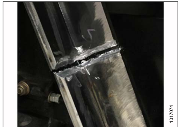
Figure 3.5: Cut in RH Brace Prepared for Welding
