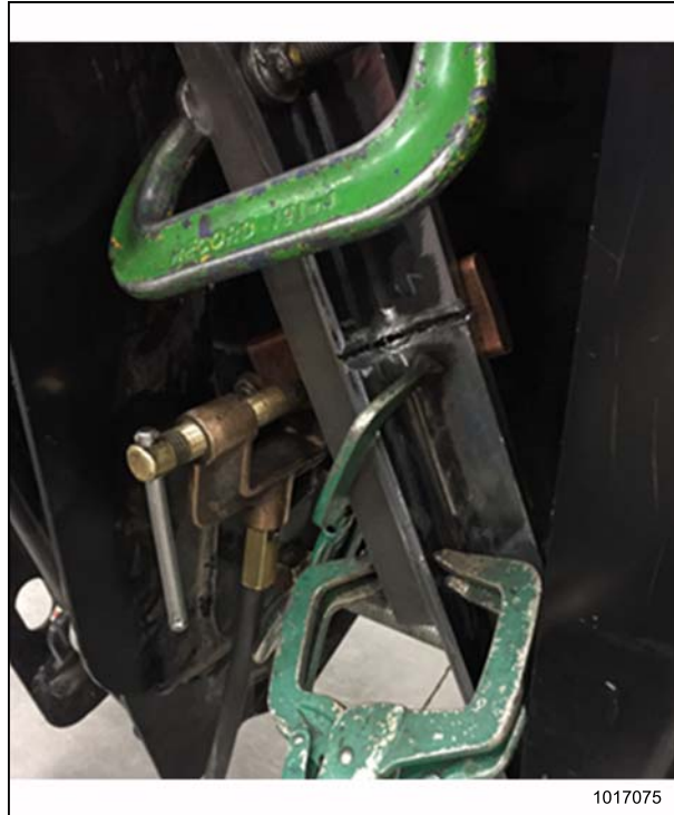
Figure 3.6: Flat Bars Clamped against Brace
