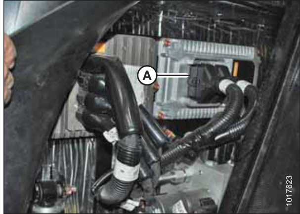
Figure 1.21: Firewall Extension Module
