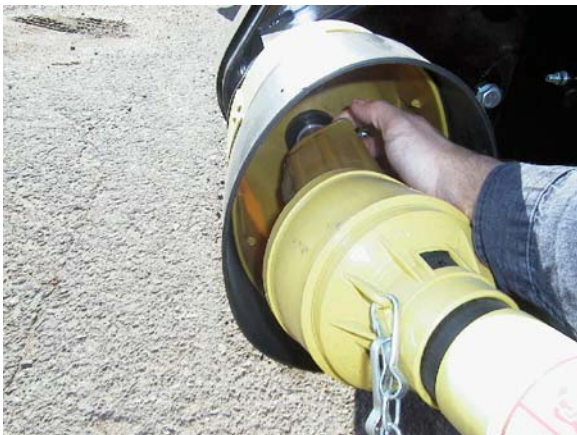
Drive Shaft to Header Installation
