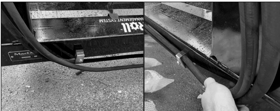
Figure 17: Re-securing RED hydraulic hoses.
