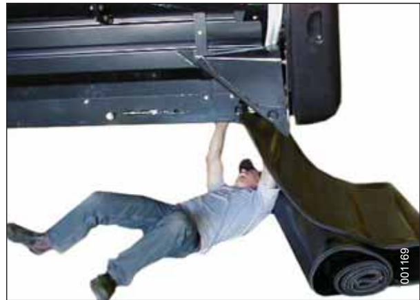
Figure 5.110: Installation du tapis
