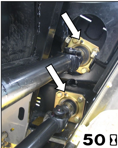
ROLL SHAFT BEARINGS (2 PLCS)
