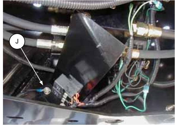
MOUNT HARNESS BLOCK ON SHIELD & ATTACH GROUND WIRE
