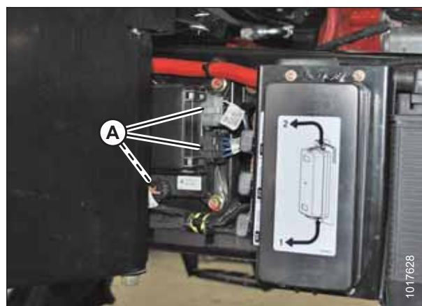
Figure 1.23: Chassis Relay Module
