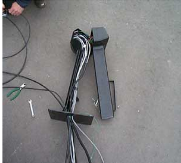
PEDESTAL READY FOR SWITCH
