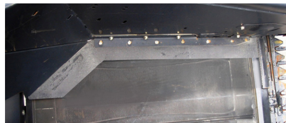
DEFLECTOR AFTER TRIMMING
